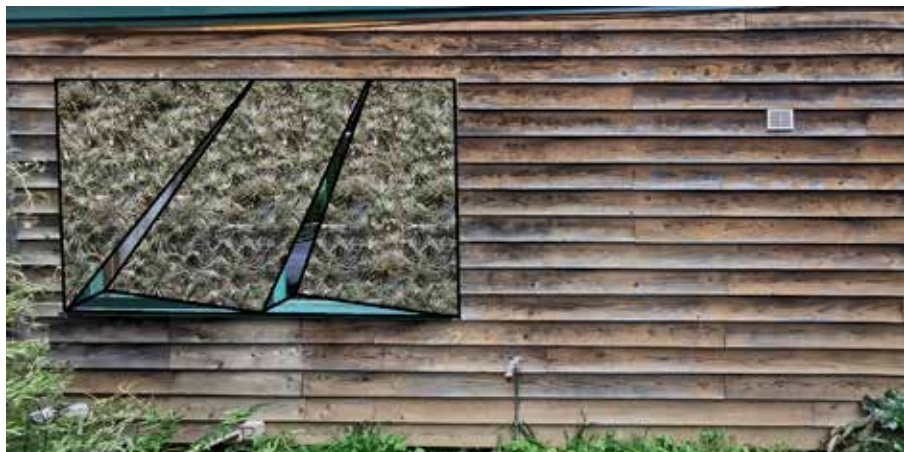
Jib screen, similar to a set of jib sails on a yacht, the screen projects outward at the bottom and the one side which allows light to enter the room from both below and from the side, but screens direct summer sun
