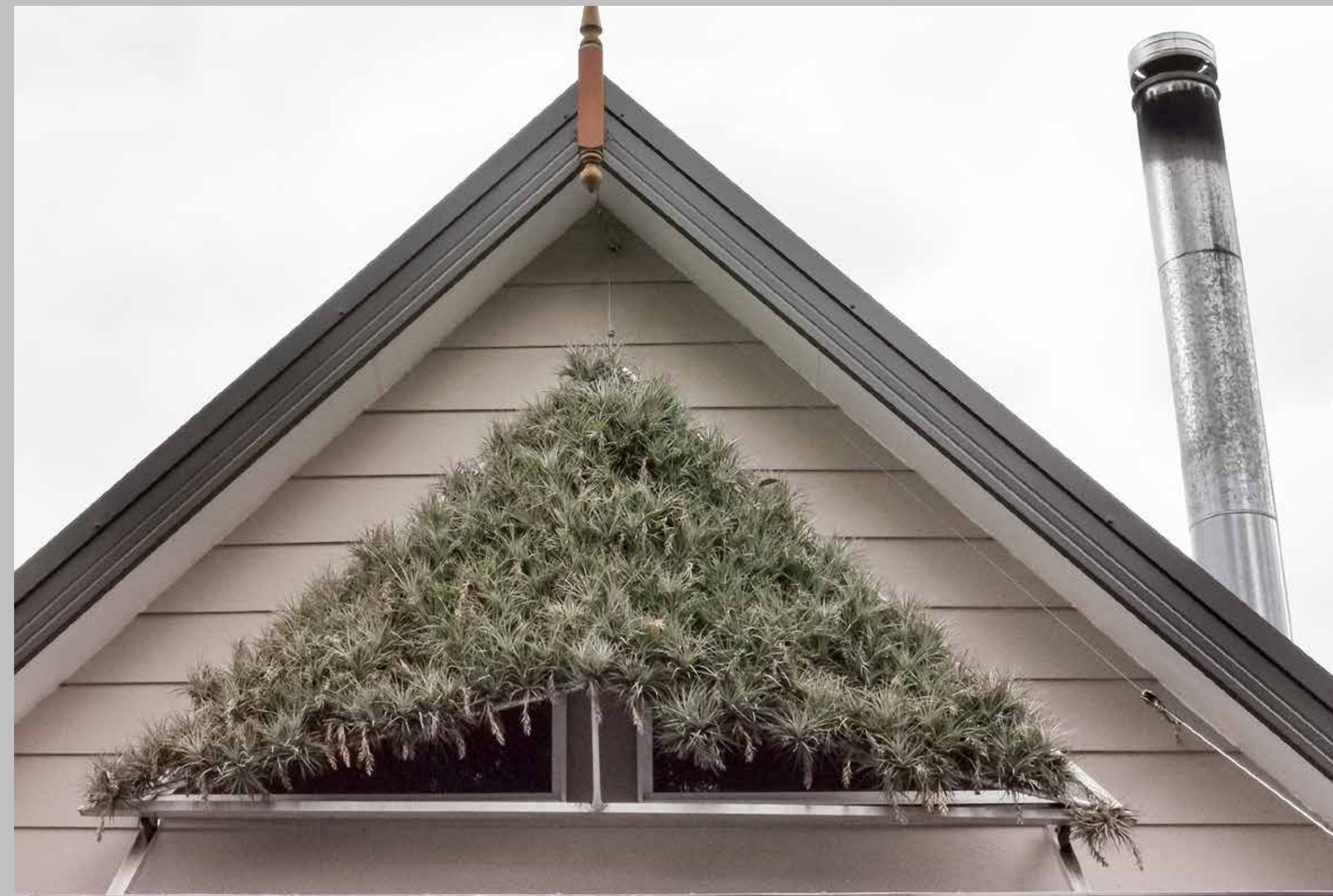
Photograph 2019 - Over three years the screen required no maintenance, and despite hot dry conditions, no plants died - the 2 photographs demonstrate the growth in the plants over this period. One plant far right bottom has slipped the mount but is still attached.
