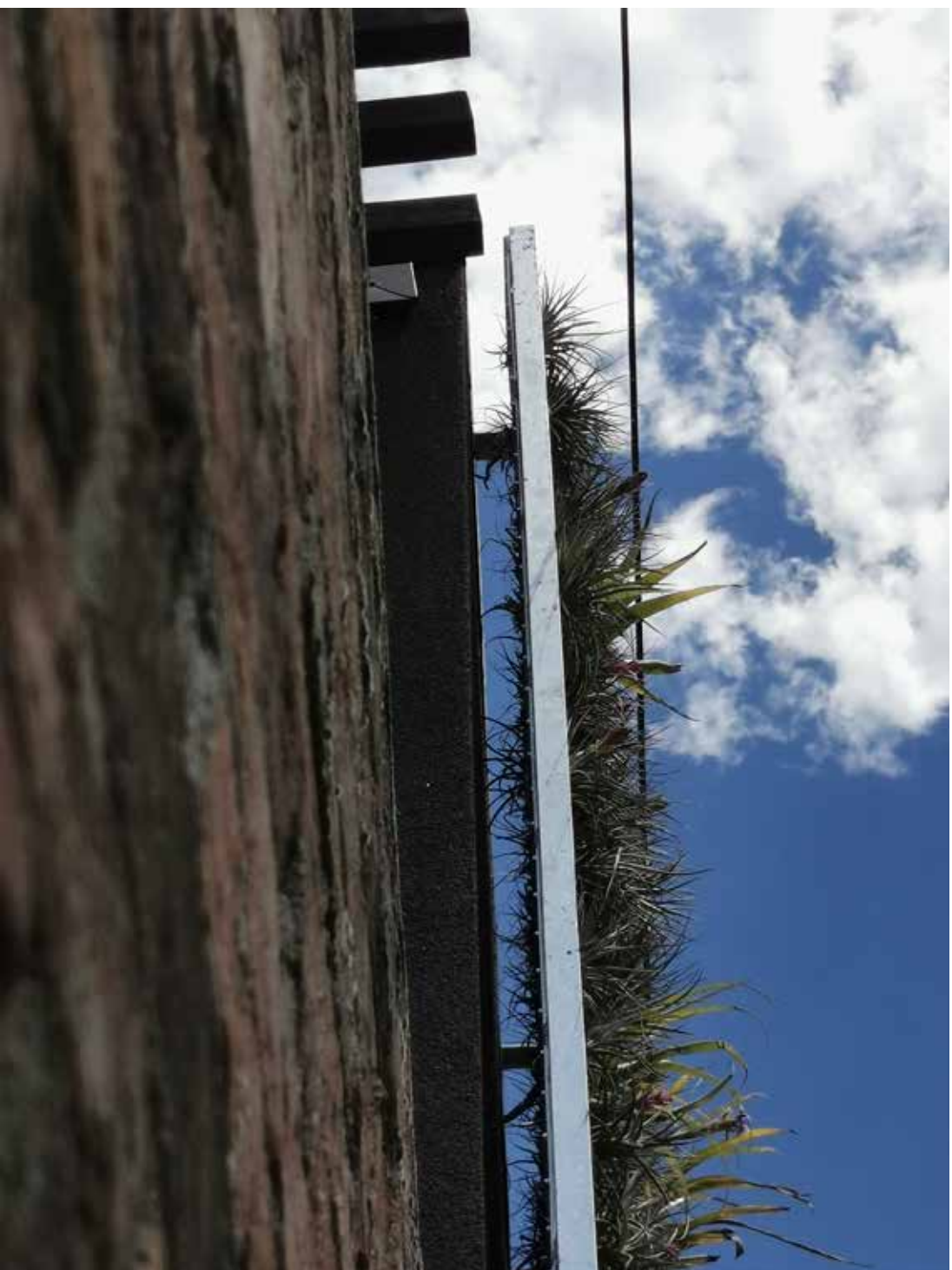
An insightful photograph of a cross section xeric tillandsia vertical wall. No plastic water proof membrane required. NO medium for roots. (many vertical gardens use compressed plastic micro fibres) NO fertilizer. NO reticulated water system. Very light weight
