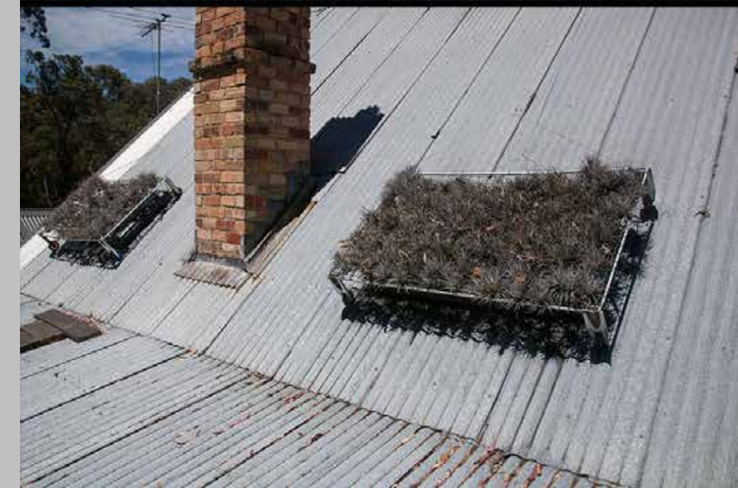
Temperature reading summer 2018 ambient air 42°C, iron roof 84.5°C, shade from Tillandsias 53.1°C - heat mitigation on iron roof of 31.4°C
