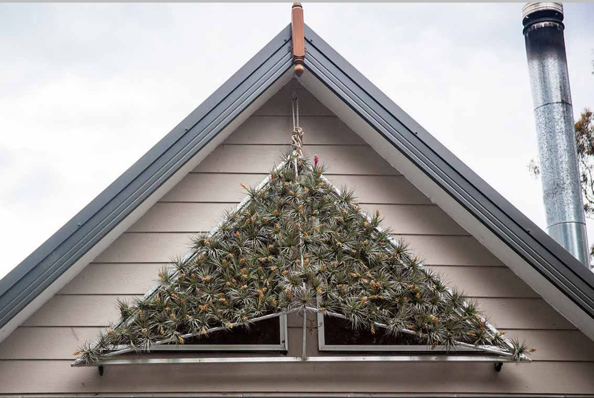
The screen is held in place during the installation before the wire cable and pulleys were installed. Notice how the screen is projected out from the wall at the bottom to allow light to enter the space. Photograph 2016
