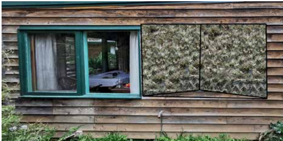
Nose screen, projects outward at the bottom which allows light to enter the room from below but screens direct
