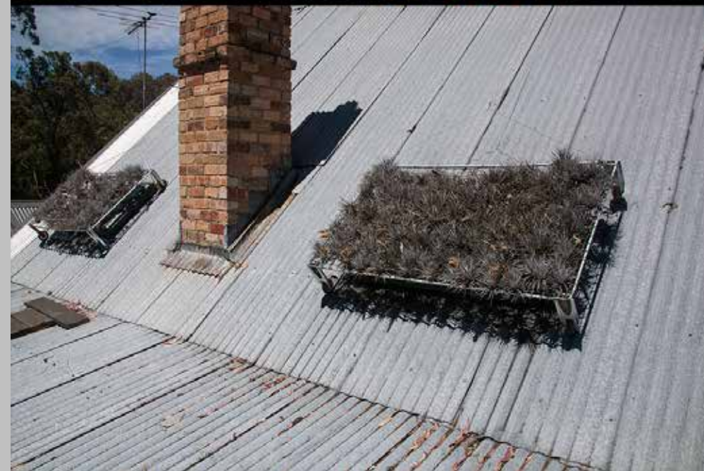
Above: the Tillandsia screens over and away from the skylights. Right: Tillandsia screen in flower.
