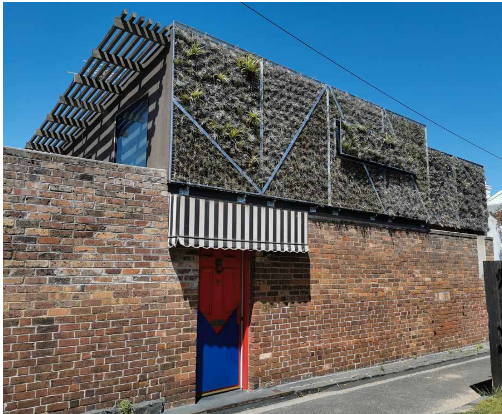
Second four panels of Tillandsia screens installed late October 2021. ( due to Covid lock down installation was dramatically delayed)
