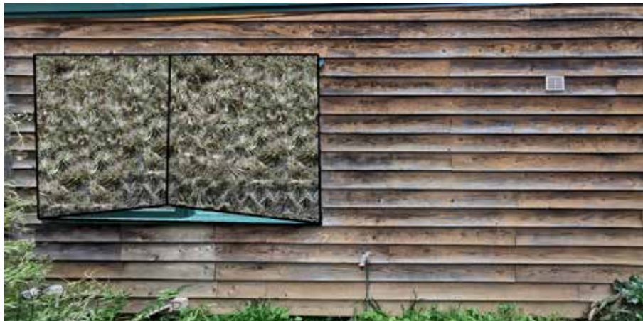
Nose screen, projects outward at the bottom which allows light to enter the room from below but screens direct
