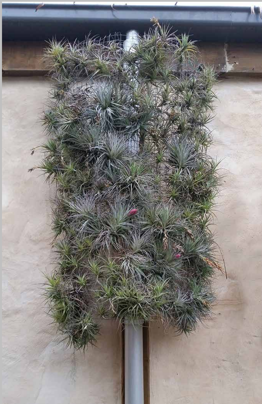
Even the most refined architecture can have awkward areas where utilitarian facilities like water and other services sit on the exterior of the facade. As this experiment shows, in this situation Tillandsias are used to screen a spouting down-pipe. When access is needed the structure supporting the Tillandsias is simply hinged away from the pipe.
