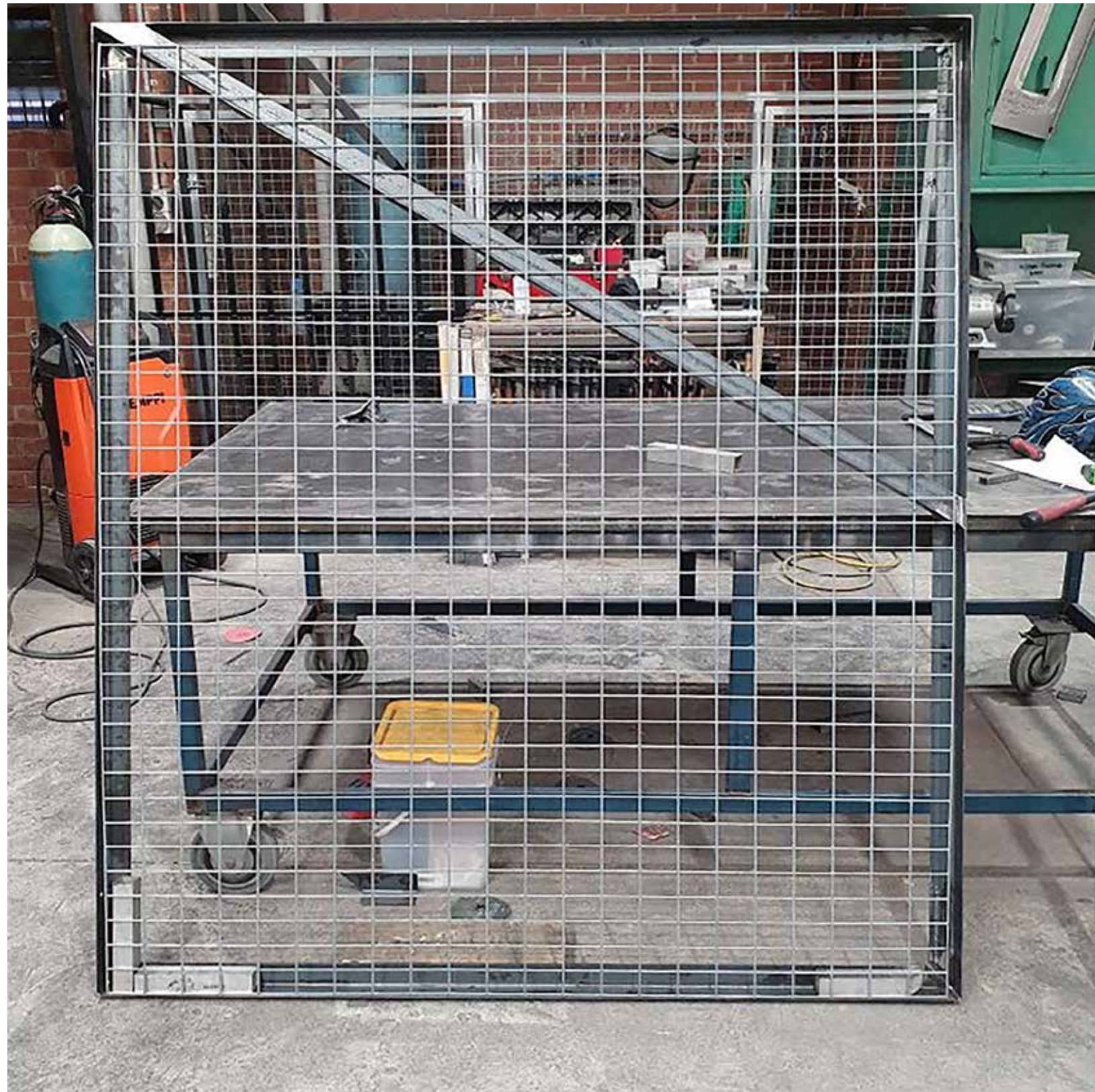
Screen fabricated and ready for hot dipping galvanized in the fabrication workshop.
