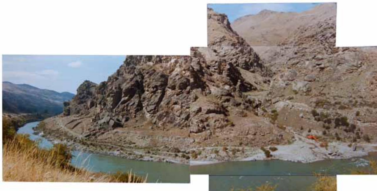
Cairnmuir face and the Clutha River 1984 notice the fruit growers road on the opposite bank of the river. This was eventually flooded when the dam was filled. On the lower left is a digger undertaking some work for the construction of the dam.
