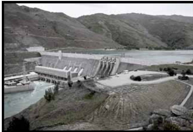
The Clyde Dam with Lake Dunstan. 2011
