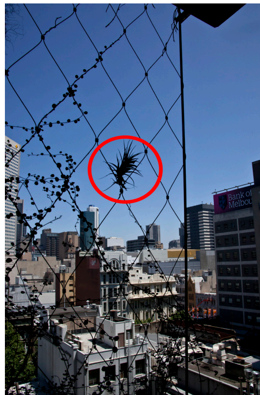
Detail of Tillandsia CH2 building North façade 2011
