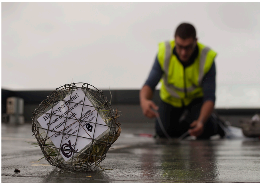
Grant Harris works in the background while the Tillandsia plant cage in the foreground is ready to be installed
