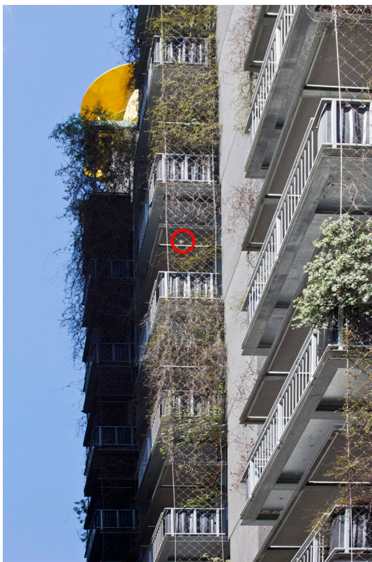
CH2 building North façade 2011. The location of the Tillandsia is marked with the red circle. Note the inconsistent growth of the climbing plants.
