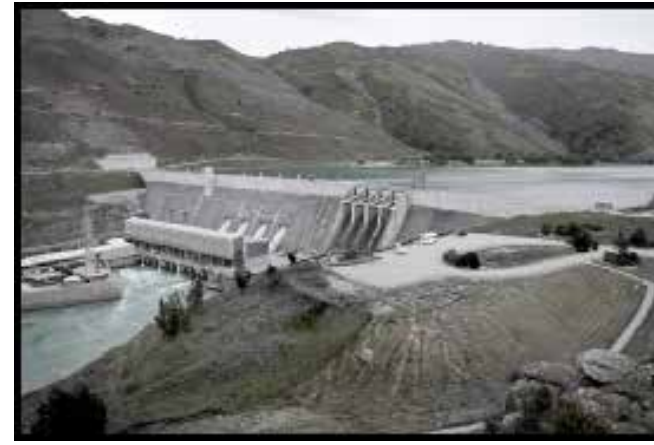
The Clyde Dam with Lake Dunstan - 2011
