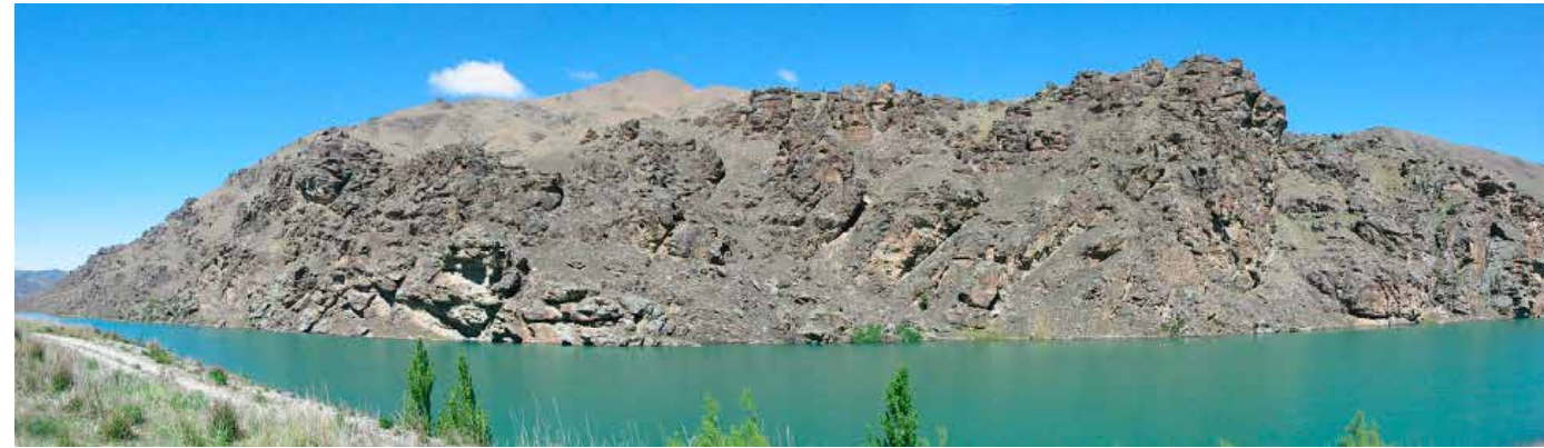
Cairnmuir face and the Clutha River after the dam fill - 2004
